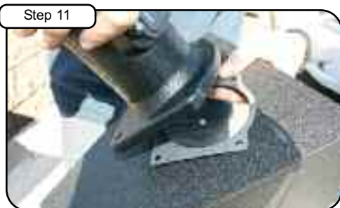
Step 11 Attach tube to outside of housing using gasket provided.
